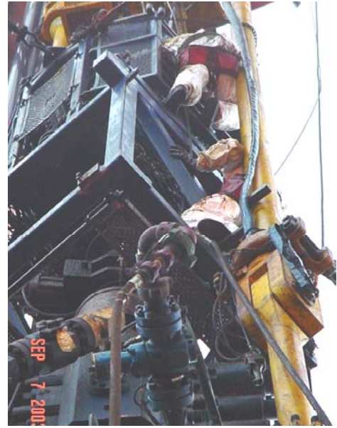
Fig. 4—CT operators trying to maneuver on a conventional tension frame
